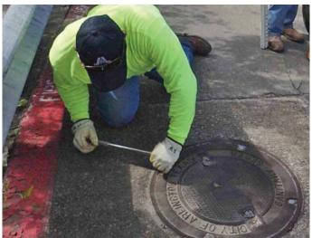
SmartCover units can be deployed easily with no confined space entry
