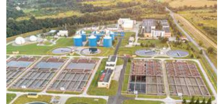
Water Treatment Plants
