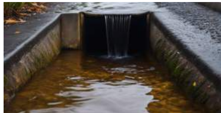
Stormwater Control Structures
