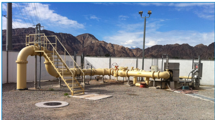
Figure 2: Primary sewage lift station in the Coachella Valley Water District
