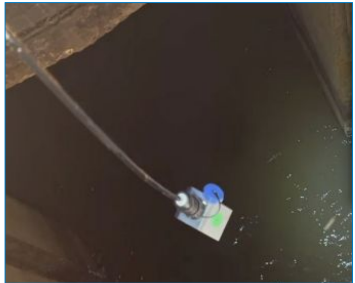
Figures 3&4: DC Water SmartCover installation
