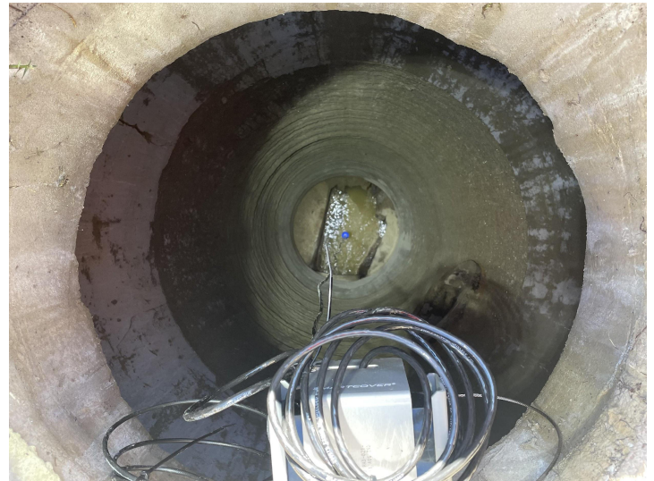
Figure 2: Side mount of the SmartCover SmartFLOE monitor
